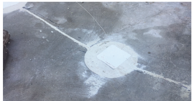
RECESSED SINGLE FIBER STAR PAD AND FILLED FIBER CHANNELS READY FOR TILE OR PLASTER APPLICATION.
