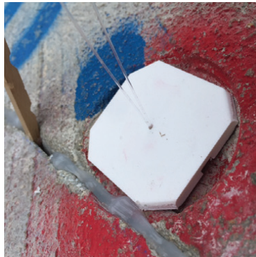
DOUBLE OR TRIPLE FIBERS WILL FIT INTO STAR PAD OPENING TO CREATE A LARGER STAR EFFECT
