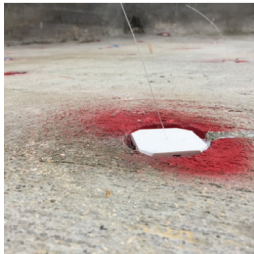
SINGLE FIBER RECESSED STAR PAD SHOWN
